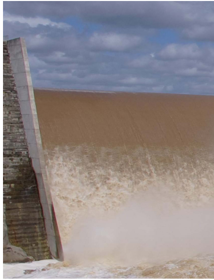
(A) Prototype scale: Paradise dam, h = 0.62 m, \theta = 57.4^\circ , d_c/h = 2.85 , q = 7.4 m 2 /s, Re = 2.9 \times 10^7 (Flow from top to bottom)
