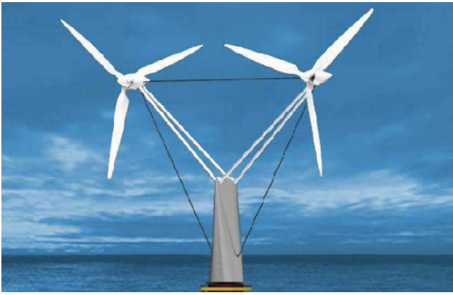
Fig. 1. SEREO structure (Herskovits et al., 2012) composed of twin wind turbines.
