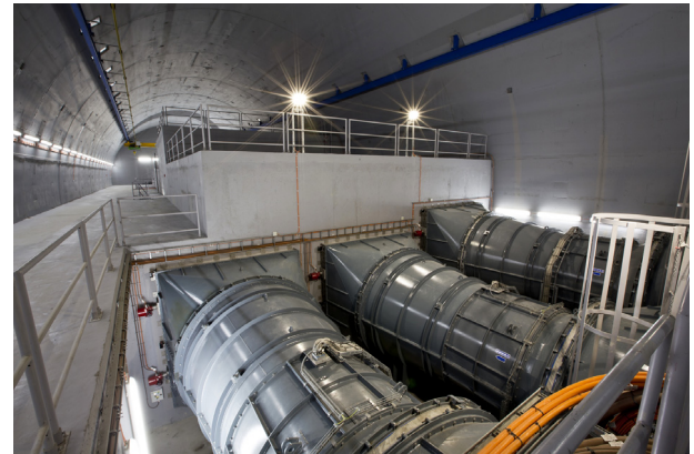
Fig. 2. Ventilation machine room Letná including three axial fans for smoke extraction from the tunnel (2015) (Karlíček, 2016; Satra s.r.o., 2017).
