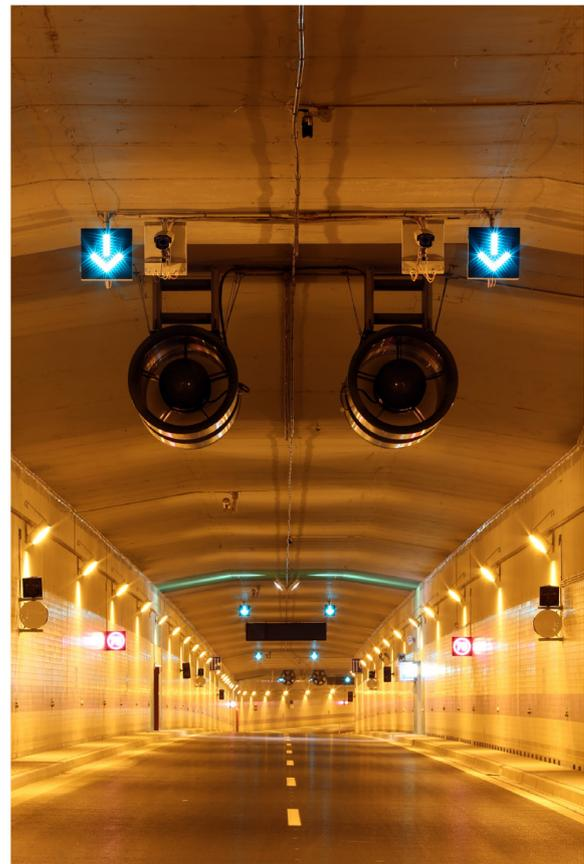
Fig. 1. A couple of jet fans located at the ceiling of the tunnel (Satra, s.r.o.; Karlíček, 2016).
