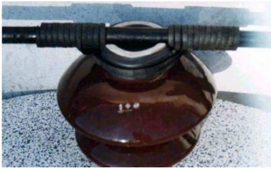
Fig. 1. Covered conductor with pin type porcelain insulator [17].
