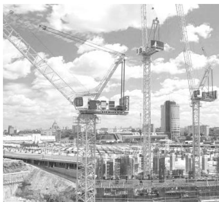
Fig. 1. Luffing Jib crane, Liebherr TurmDrehKran, (2006)
