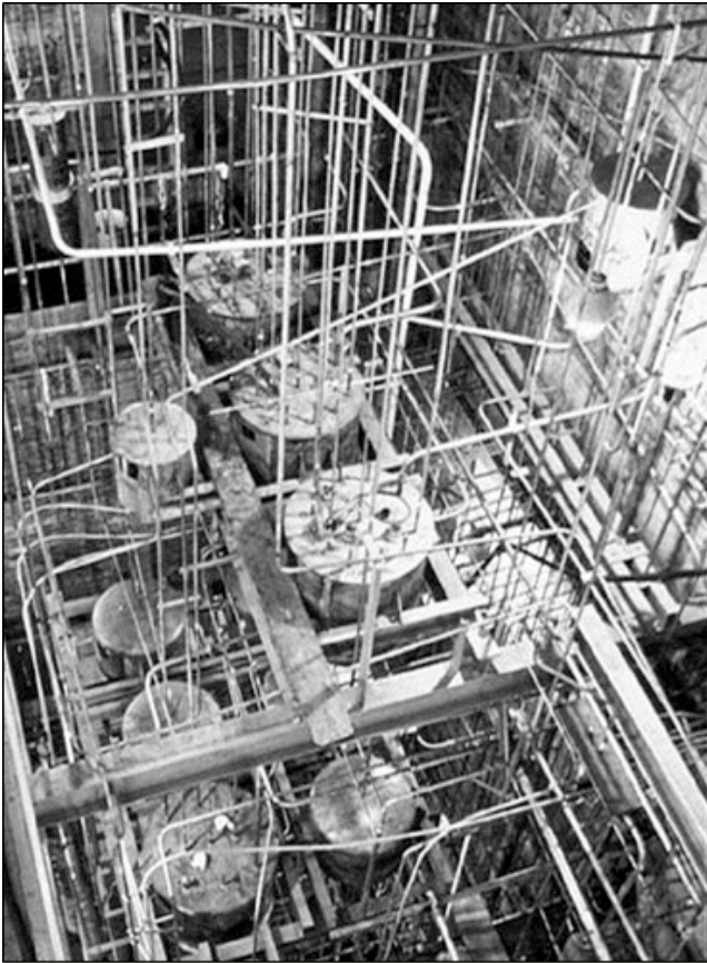
Fig. 1. Shows the nuclear cave environment, which poses a difficult characterisation task for decommissioning.
