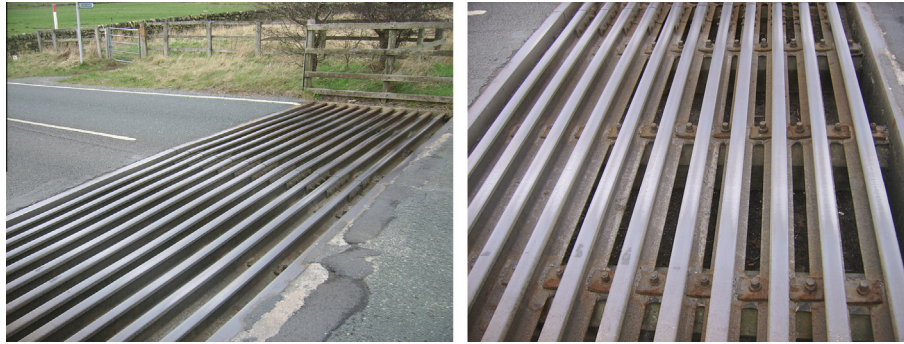
Fig. 1. Cattle grid installation on Baildon Moor (site Baildon B).
