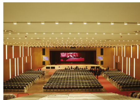
(b) The ceiling is sand panels
