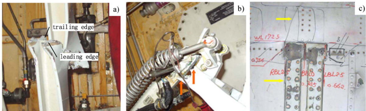
Fig. 2. Details of the fractured structures of nose landing gear: (a) down drag; (b) lock link; (c) aft bulkhead.
