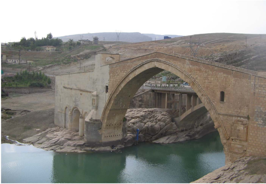
Fig. 1. View of the Malabadi bridge.
