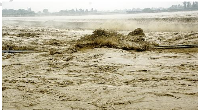
Figure 1. Lanzhou-Chengdu-Chongqing Products Pipeline floating owing to the flood scouring
