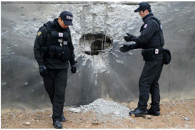
Fig. 1. Punching shear failure of concrete structures under high strain rates [7].
