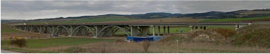
Fig. 1. General view of the bridge structure.
