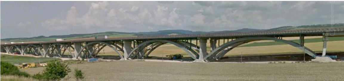
Fig. 2. View of steel bridge arch.
