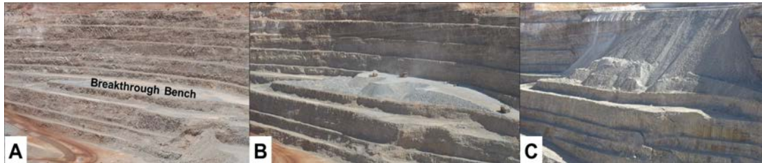
Fig. 1. Preparations for Cave Breakthrough Bench (a) Breakthrough bench & high wall in 2008; (b) Commencement of backfilling to buttress high wall in February 2009; (c) Completion of backfill buttress in October 2009 and initial cave breakthrough (cracking) observed on slope below breakthrough bench.
