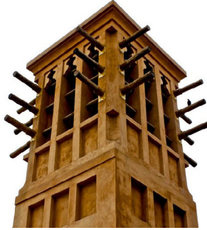
Fig. 1. Ventilation ducts - traditional Arabic architectural signs
