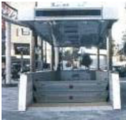
Fig. 1. Water Stop Plate.
