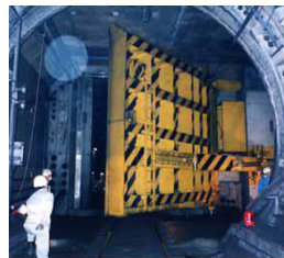
Fig. 3. Watertight Gate.
