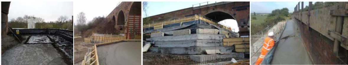
Fig. 1. Views of preparation of the underlay, a poured layer of foam concrete, the pyramidal formwork and application of the last layer of foam concrete, [5].
