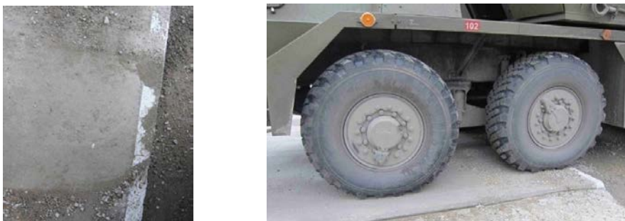
Fig. 1. Experimental application of LFC in pavements of access roads and car parks (view on top and side) in Trenčín, Slovakia [1].
