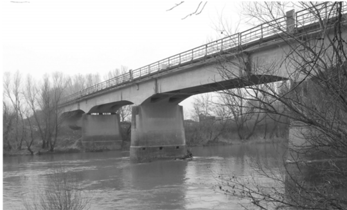
Fig. 1. View from downstream
