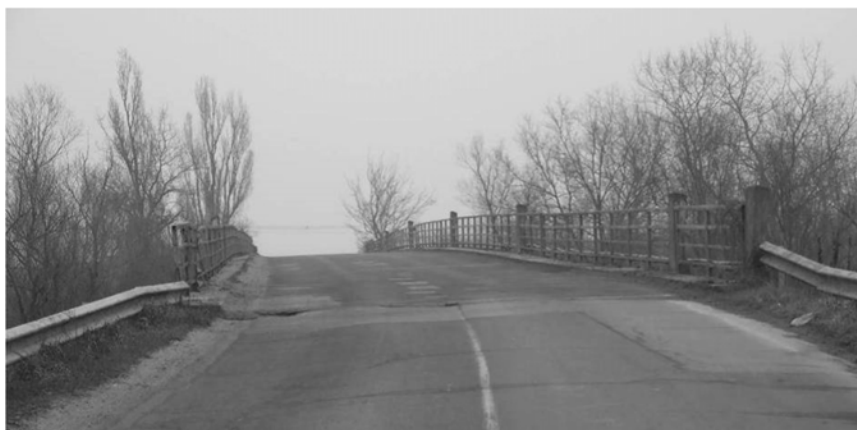
Fig. 2. Gauge of the old bridge
