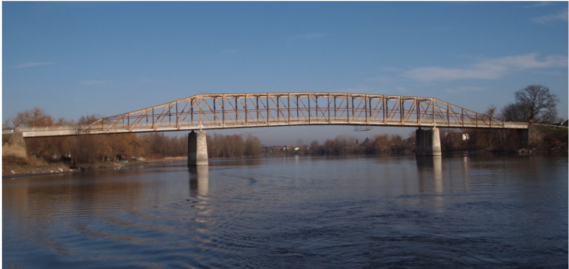
Fig. 1. Appearance of road steel bridge in Morovic
