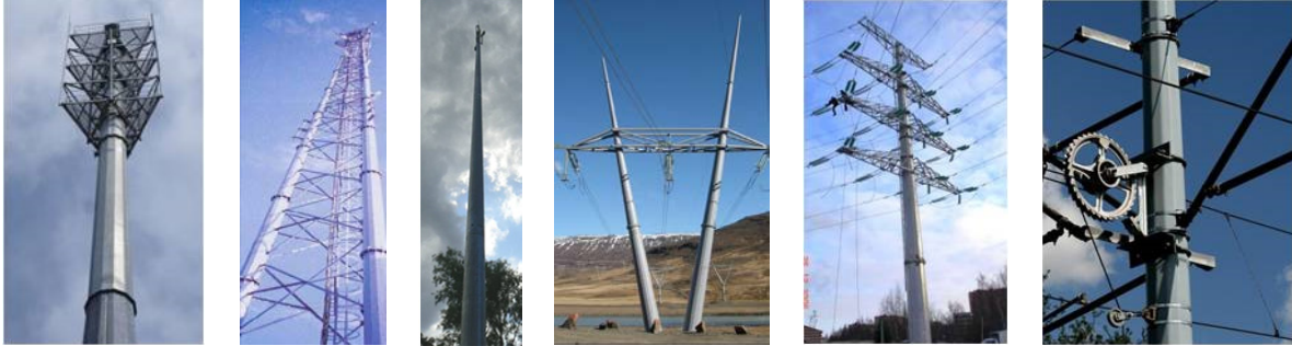
Fig.1. General design diagram of MMBC and their structures: a-c) mobile communication towers; d, e) anchor post VL 420kV; f) railway contact network support
