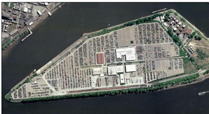
Fig. 1. Carport terminal in Hamburg harbor (Google maps, 2011_07_09).
