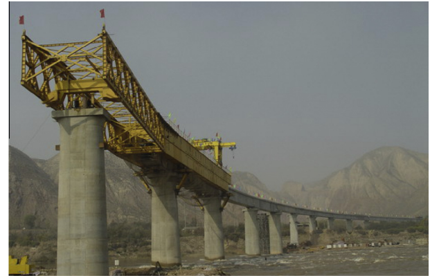
Fig. 2. A continuous curved in-plan railway bridge of the Lan-wu line, in China. (Image CC from CRCC [44]).
