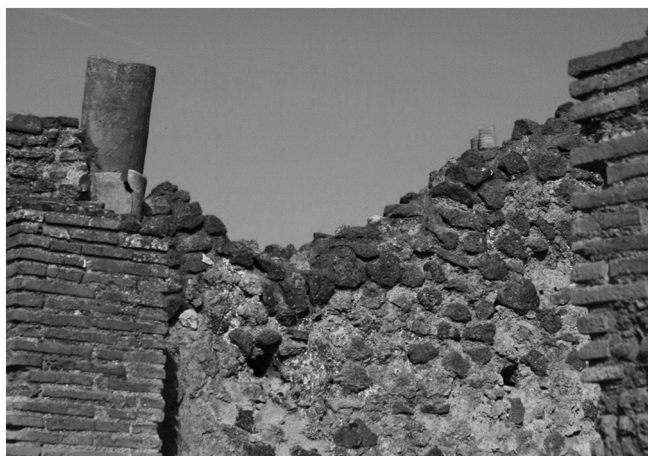
Fig. 1. Wide-bore downpipe in VI.14.7 with two narrow-bore water pipes visible in the adjoining property (VI.14.6).
