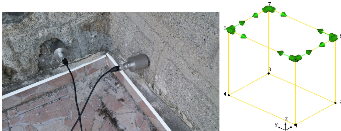
Fig. 2. The accelerometers connections and locations on the bastion.
