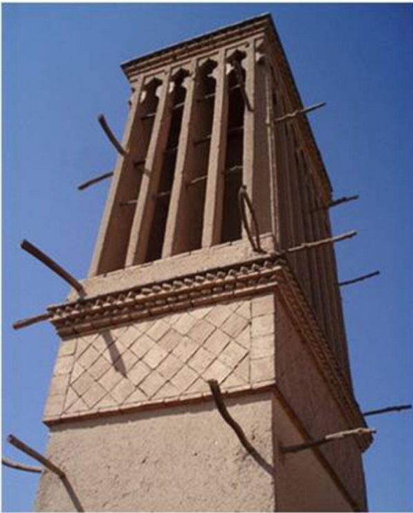
Fig. 1. A four-sided wind catcher with rectangle cross section.
