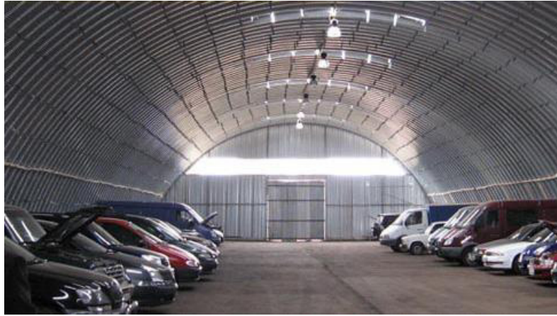
Fig. 1. Hangar for parking and repair of vehicles.
