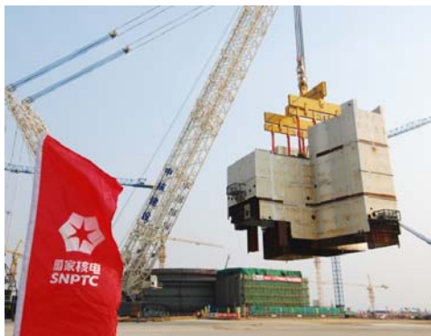
Fig.1. lifting work of CA01 module
