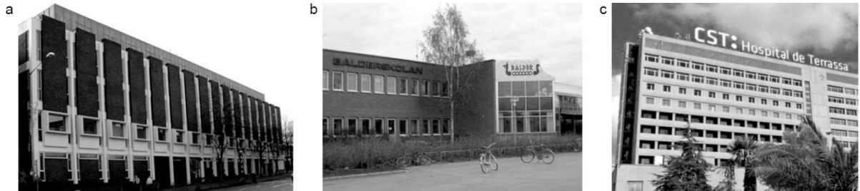
Fig. 1. (a) University Building in the United Kingdom; (b) Secondary School in Sweden; (c) Hospital Building in Spain.
