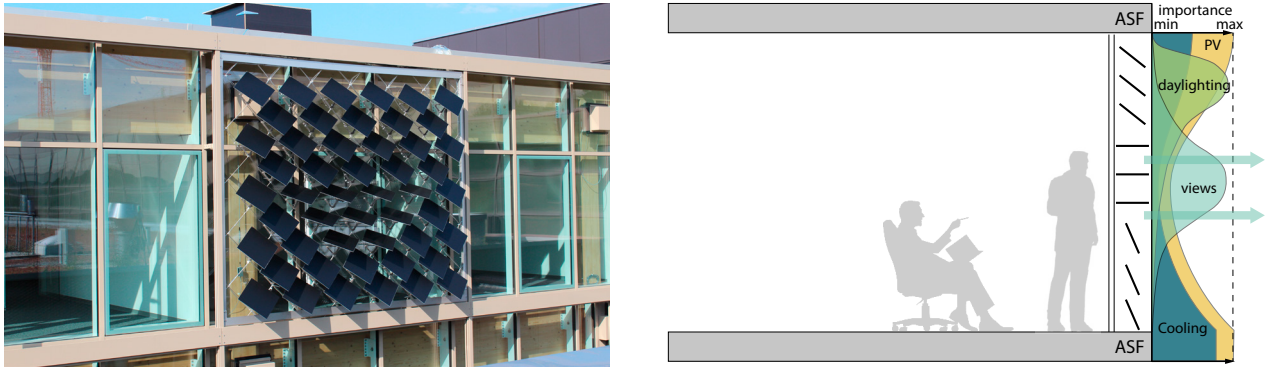
Fig. 1: Left: An example of an ASF constructed at the House of Natural Resources. Right: a schematic describing how the facade can mediate solar radiation to optimise the internal environmental conditions [6]
