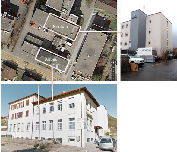
Fig. 1: Aerial (top left) and side views of the Altbau (bottom) and Neubau (right) parts of the Sargans building
