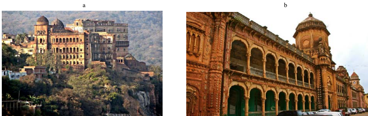
Fig. 1. (a) View of Mubarak Mandi Campus; (b) Front Façade of Army head Quarter
