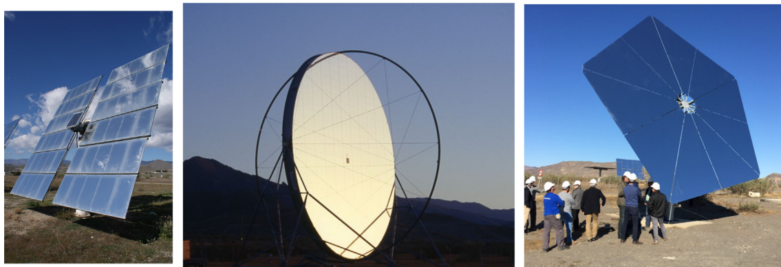
Fig. 1. Heliostat types: T-Type (left), ASM 150 stretched membrane (centre), Pentagonal slope drive 'Stellio' (right).
