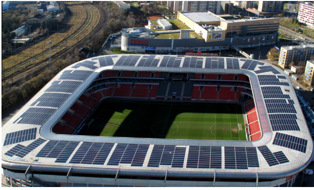
Fig. 1. The birds eye view of the building integrated PV power plant on the roof of the football stadium.
