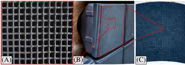
**Fig. 1.** The receiver of the solar tower Juelich. (A) shows a close up of the absorber structure of the Hitrec-II absorber module, (B) individual absorber modules during maintenance which make up the main receiver of the solar tower Juelich (C).
