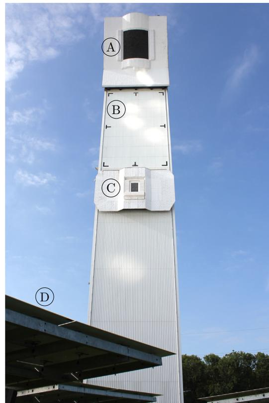
**Fig. 3.** Photo of the STJ displaying the main receiver (A) at the top, the target for the calibration of heliostats (B), the Testreceiver (C) and the heliostats (D) at ground level.
