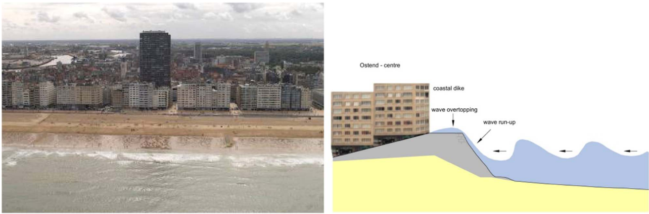
Fig. 1. Ostende, a city along the Belgian coastline, has the waterfront close to its apartment buildings (pictures: Masterplan Coastal Safety Belgium – Flemish Government – Coastal Division).
