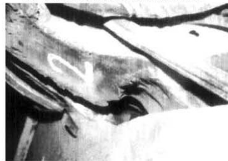
(c) Erosion in guide vane portion
