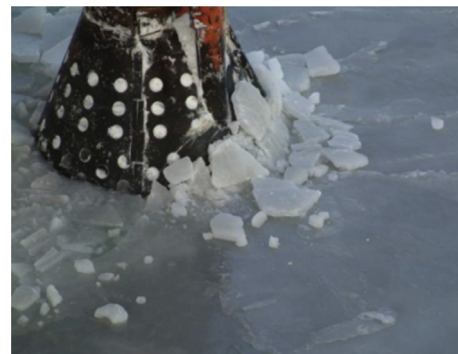
Fig. 2. Ice-breaking cone on jacket leg in Bohai Bay.
