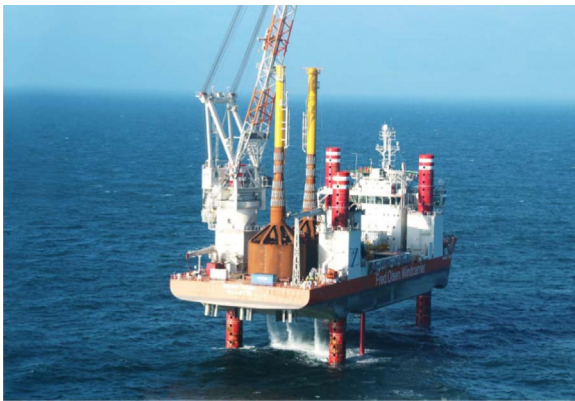
Fig. 2. Prototype Bucket foundation prior to installation.
