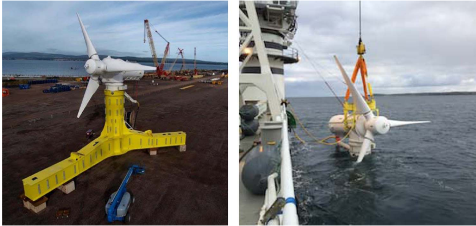
Fig. 1-1. Andritz Hydro Hammerfest 1.5 MW rated TST with installation into the Pentland Firth, Scotland (images credit: Atlantis Resources Ltd.) as part of the MeyGen Phase 1A deployment.
