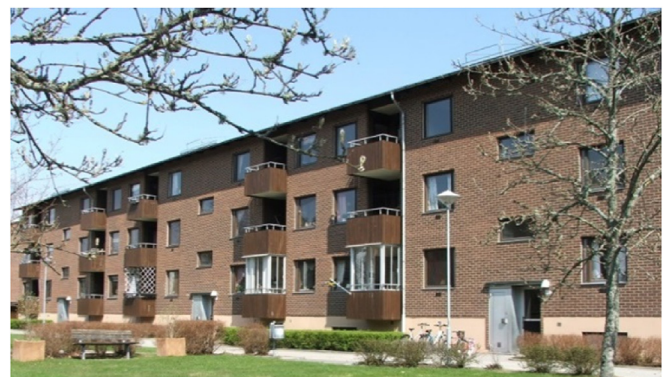
Fig. 1. The case-study concrete-frame building in Ronneby, Sweden.
