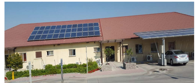
Fig. 1. The First 8.64 kW BIPV at Sadeem building in Bapco at Awali, kingdom of Bahrain.
