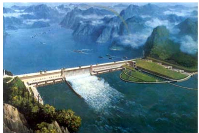
Fig. 1. Three Gorges power station.
