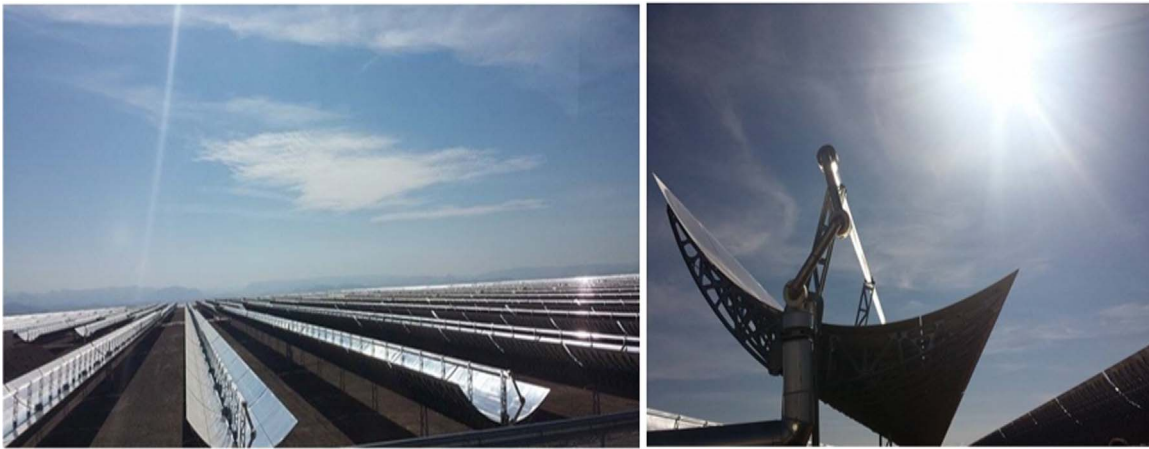
Fig. 1. Concentrated solar power using a parabolic trough collector: 160 MW power plant, Noor I in Ouarzazate solar complex, Morocco.
