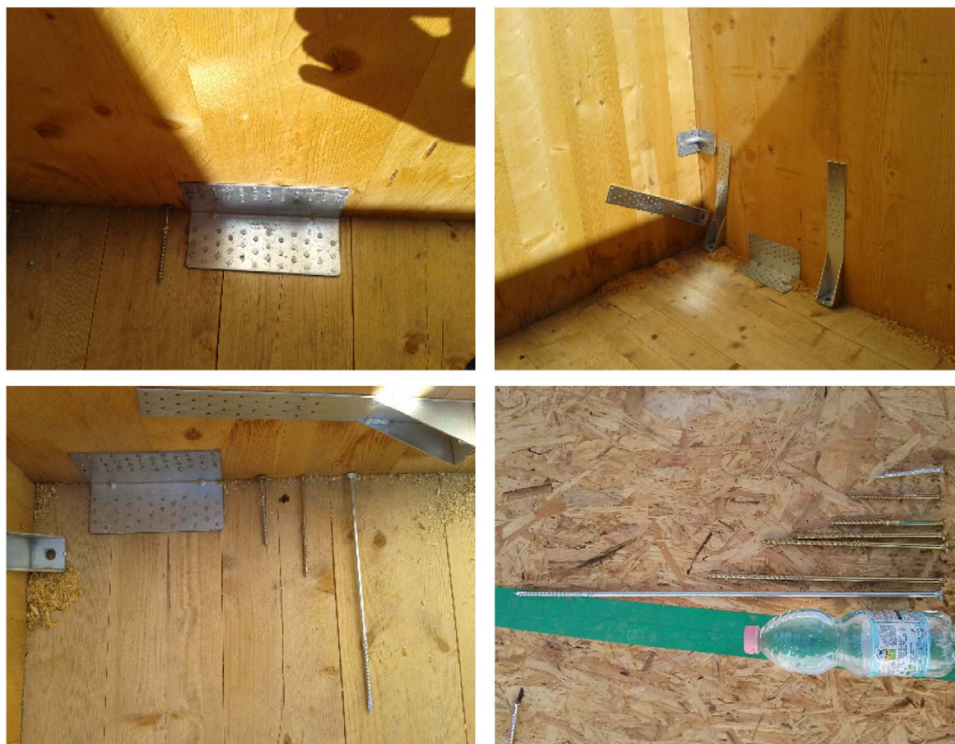
Fig. 2. different types of screws, joints and junctions used with precast timber panels. Pictures from different building constructions.
