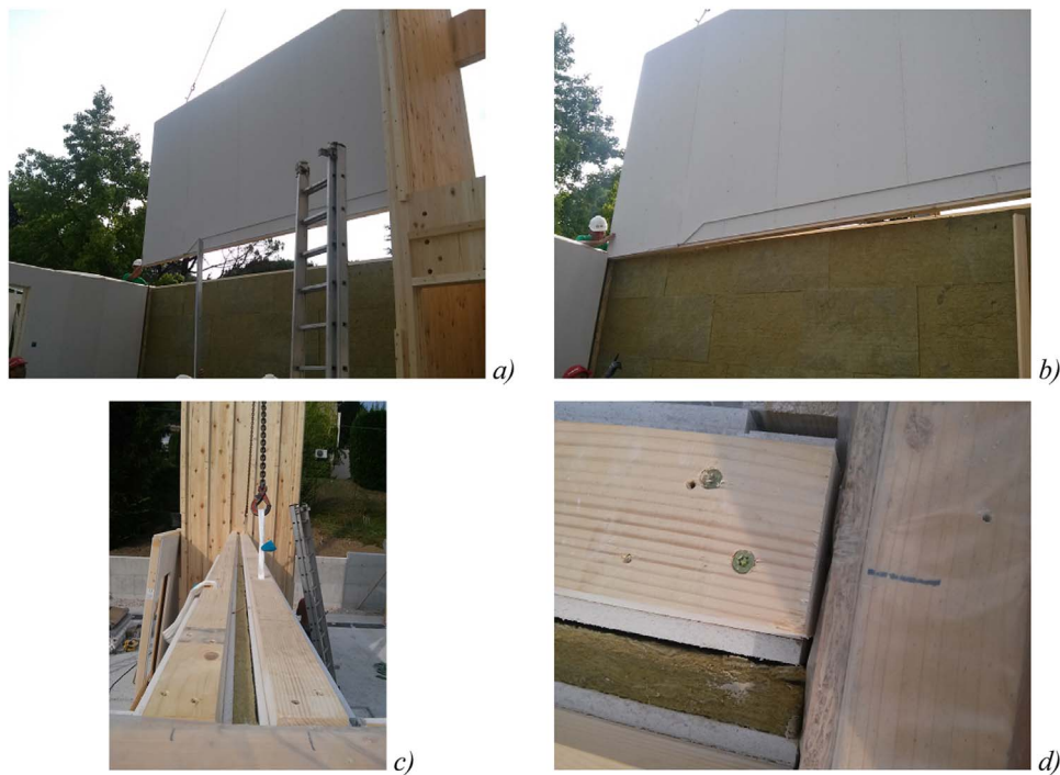
Fig. 1. Example of wall assembling in a multi-storey light weight timber building. From a) to c) the panel is let down using crane. In d) the high requested precision and accuracy is highlighted.
