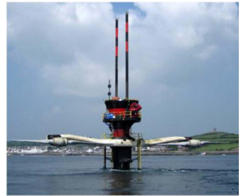
Fig. 3. The 1.2 MW SeaGen tidal energy system (UK). Adapted from [11].
