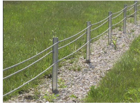
Fig. 1. Three-strand CMB. ( http://safety.fhwa.dot.gov/roadway_dept/policy_guide/road_hardware/resource_charts/cable.pdf ).
