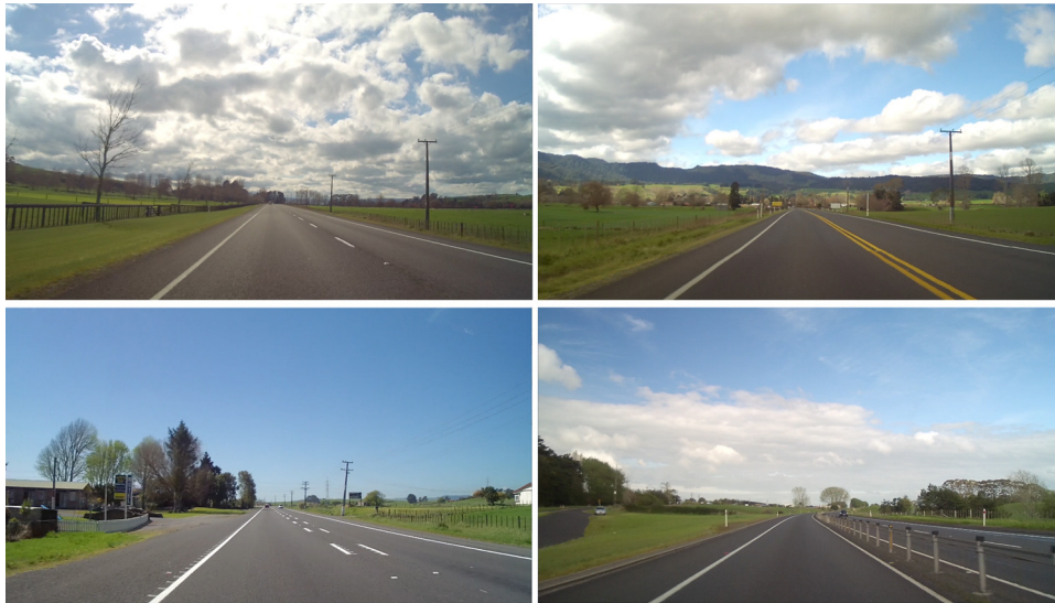
Fig. 1. The four median treatments selected for testing. Clockwise from top left: Dashed white control, double yellow, wire rope barrier, wide centreline. (For interpretation of the references to colour in this figure legend, the reader is referred to the web version of this article.)
