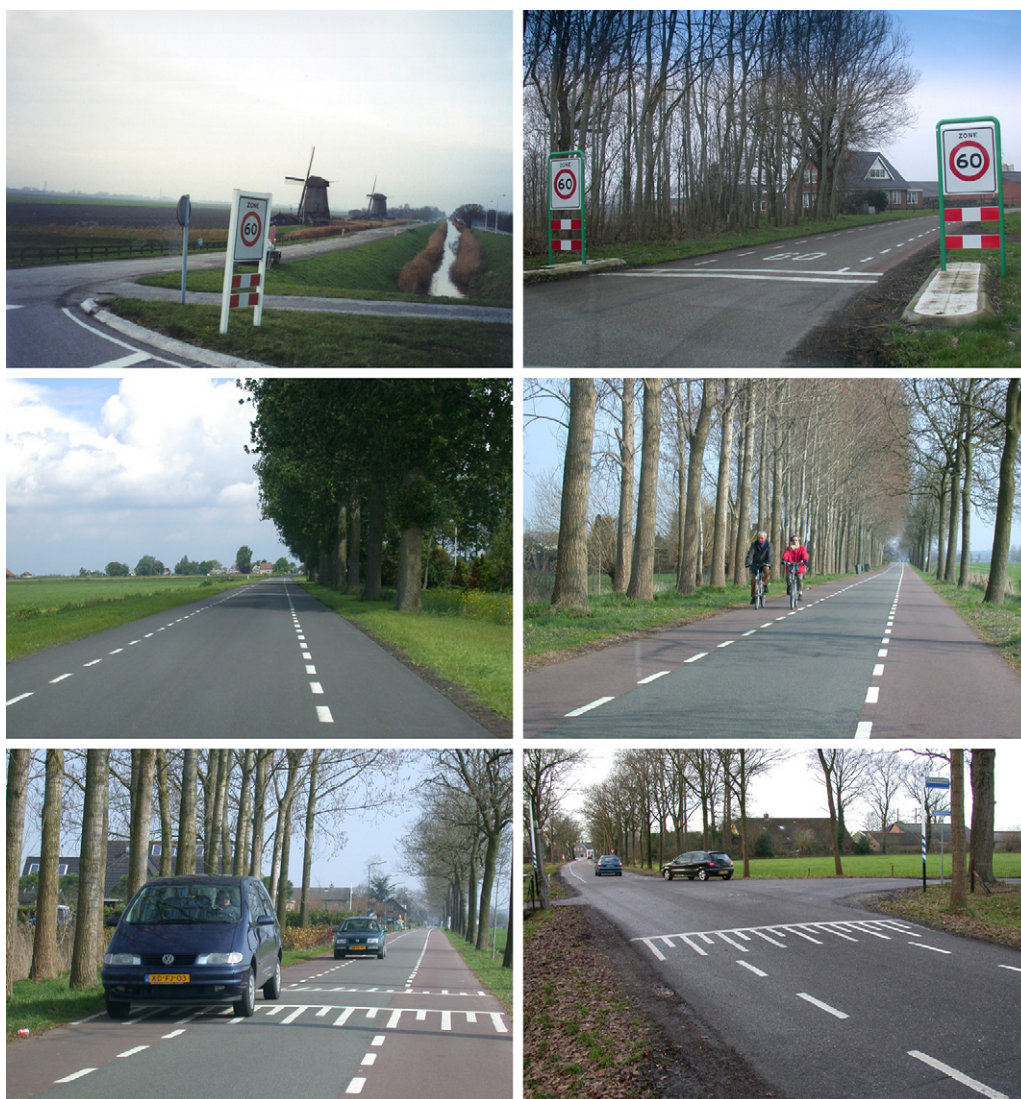
Fig. 1. Illustration of technical interventions with a low cost design. Zone-boards with double stripe (above), edge markings instead of central markings (centre left) and red-painted, non-compulsory bicycle lanes (centre right), speed hump at road segment (lower left) and raised level at intersection (lower right). (For interpretation of the references to color in this figure legend, the reader is referred to the web version of this article.)
